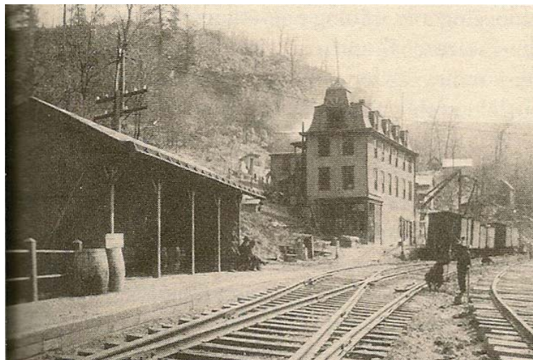
The railroad depot at Bear Run in the 1890s, with a rather sad, barren hillside in the background. (Toker 87)
